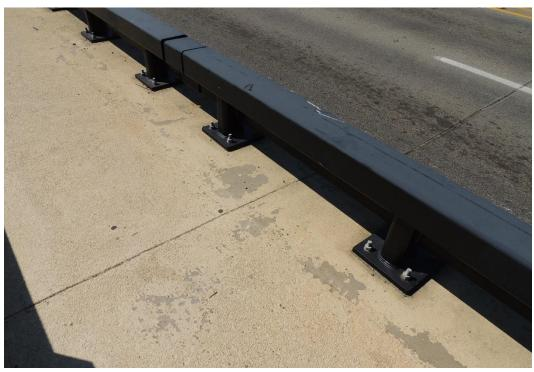
Condition Photo 17: Vehicular scratches/damage to the metal curb rails on the sidewalk.
