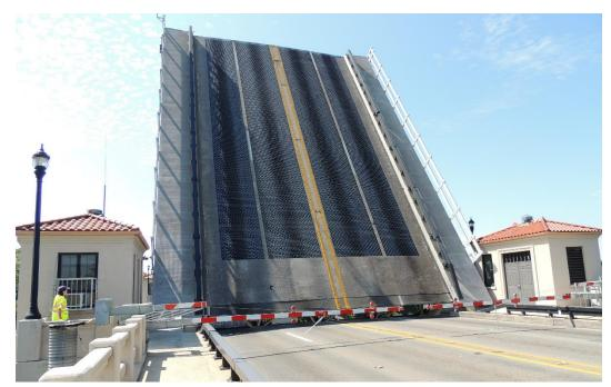
Condition Photo 10: The east side of the bascule span in the lift position and the traffic gates, looking west.
