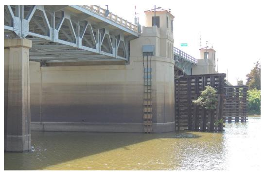
Condition Photo 28: Pier 5 of the bascule span and vegetation growth in the east timber fender system.
