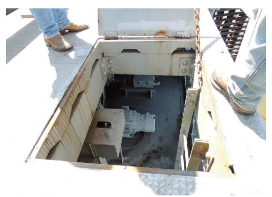
Condition Photo 18: The gearing and equipment for the locking system for the bascule spans housed under the sidewalk.
